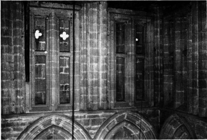
Square grids, dating from about 1356, in the central tower. They were inserted to stabilise the structure.
