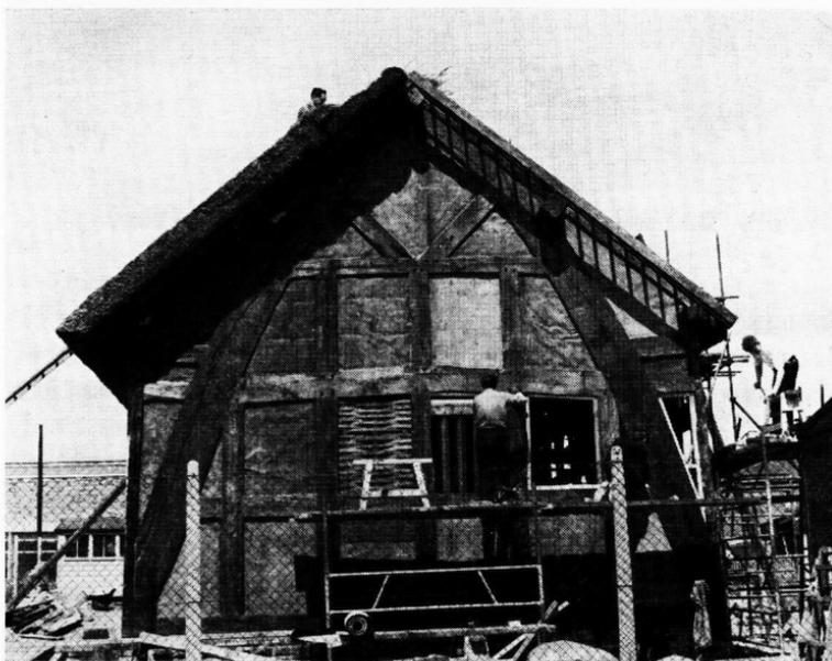
PLATE III. Newton Hall: the south gable end, showing a typical window and a wattle panel woven with riven oak laths.
