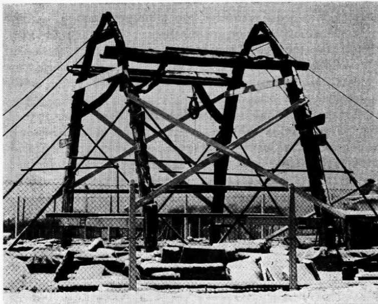
PLATE II. *Newton Hall*: the centre pair of cruck-blades after the removal of the oak frame walls and roof.
