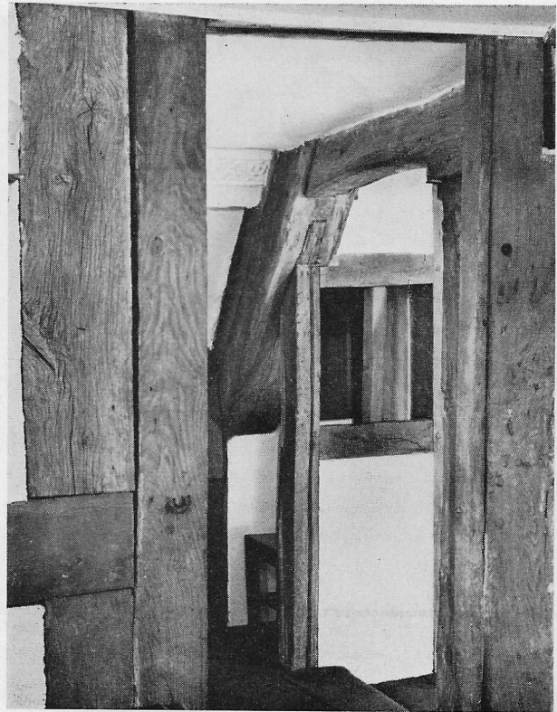
FIG. 13. Confessional in Oratory on second floor.
