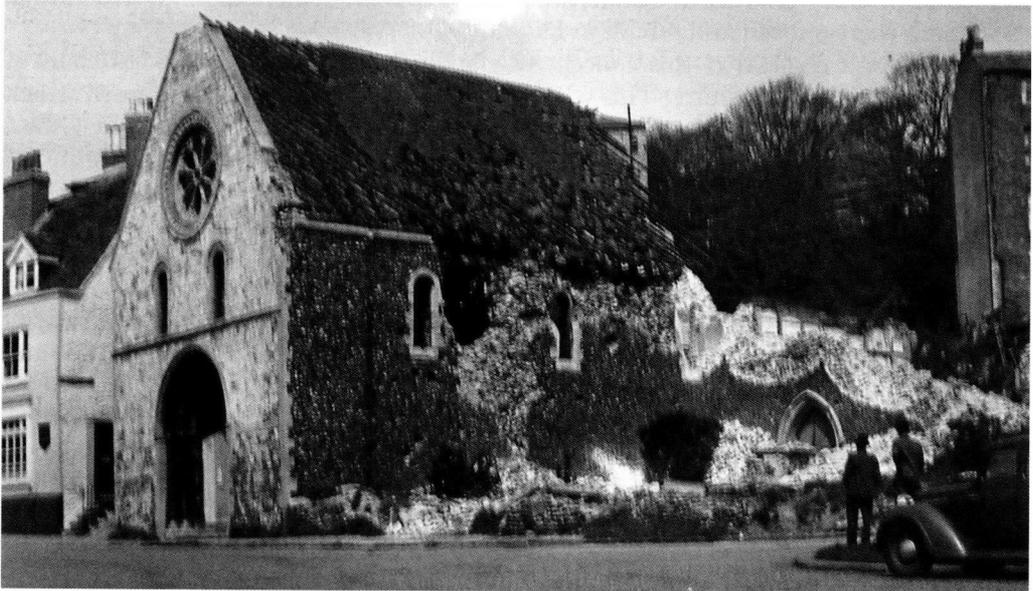
Fig. 7. St James, Dover, 9 May 1950, after collapse of war-damaged tower.
