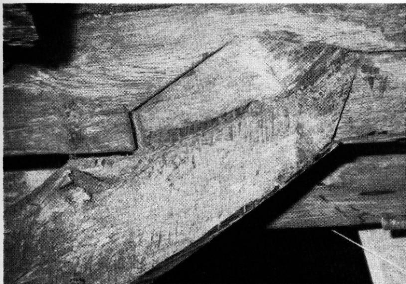
FIG. 8. The lower of the two notched-laps in the belfry, here designed to withstand mainly compression, but also notched to resist any tendency to withdrawal.
