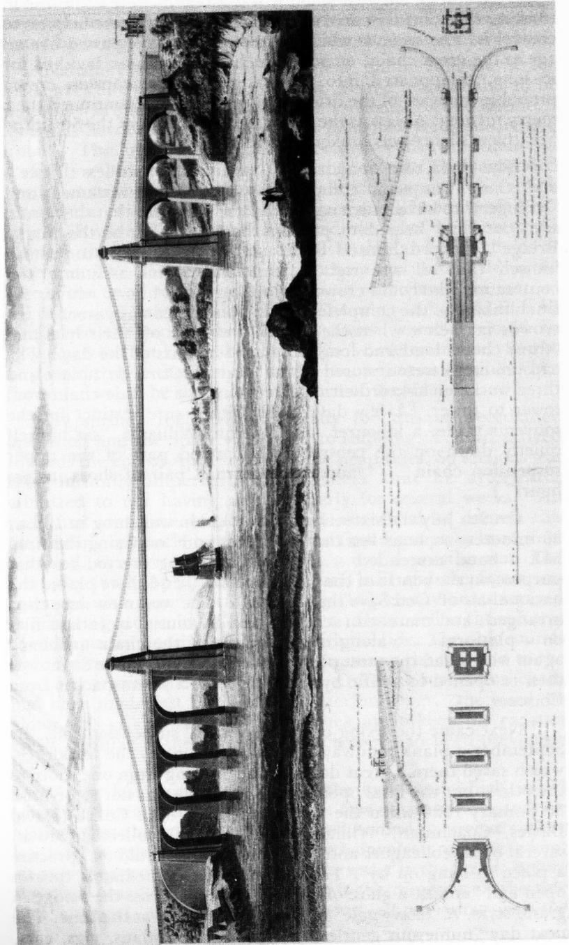
*Suspension Bridge over the Menai Straits between the County of Carnarvon and Island of Anglesey (plate 70, from the Life of Thomas Telford (Atlas) by himself). The section shows the method of securing the chains.*
