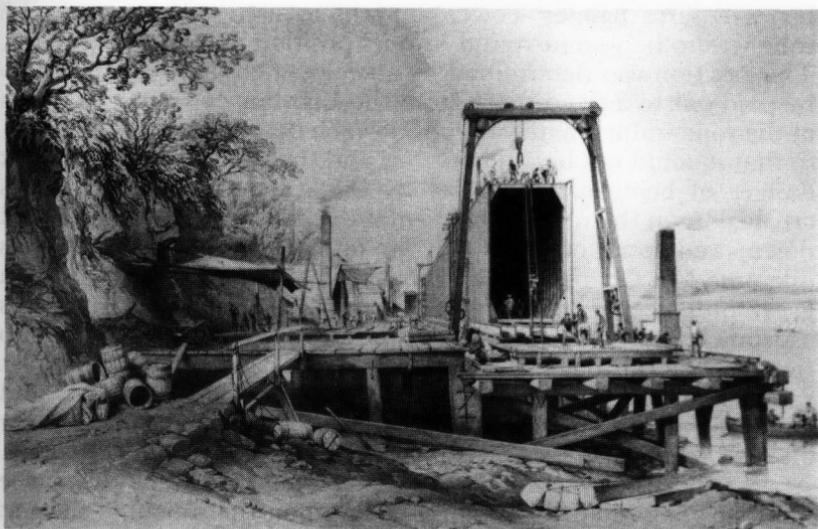
Britannia Bridge. Platform & construction of the tubes, September 1848.
