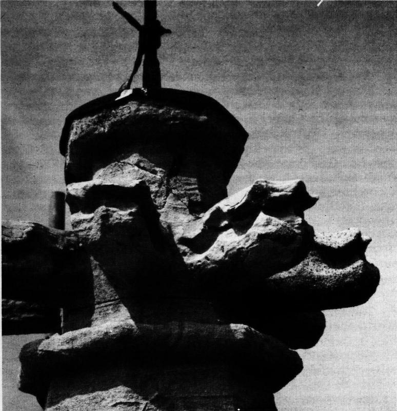
Pinnacle showing stone decay and the effect of old plastic stone repair.
